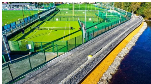
Dodder Greenway & Flood Defence Herbert Park to Donnybrook – aerial view
